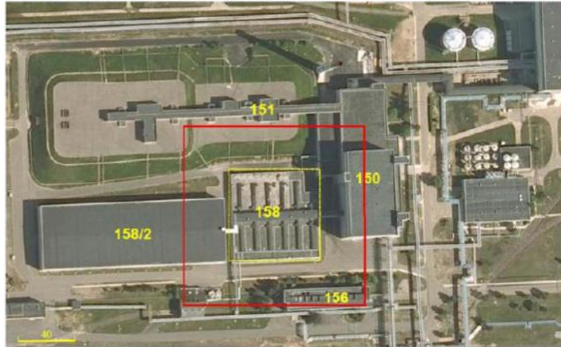
Figure 3. Reconstruction of bituminized radioactive waste storage facility (Building 158) into a repository. The red line marks the 36 m wide area around the building that will be used for the engineered barrier
