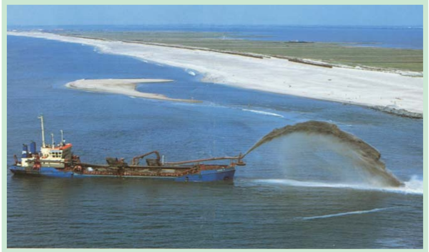
Sand spill into Baltic Sea near-shore
