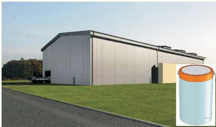
General view of spent nuclear fuel storage facility. 202 CONSTOR RBMK1500M/2 containers will be placed inside (height of container approximately 4.5 m, diameter – approximately 2.7 m). Operational time – not less than 50 years
