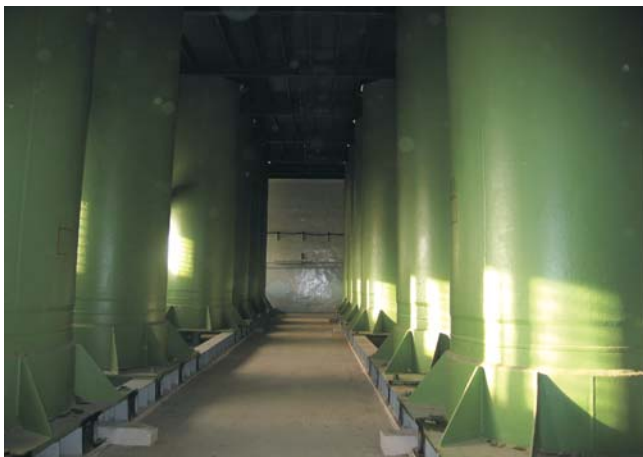
During the implementation of the project, full documentation for reactor emergency cooling system cylinders and other Ignalina NPP 117 / 1 building equipment dismantling and decontamination was prepared
