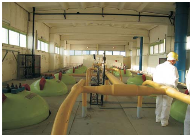
During the implementation of the project, full documentation for reactor emergency cooling system cylinders and other Ignalina NPP 117 / 1 building equipment dismantling and decontamination was prepared
