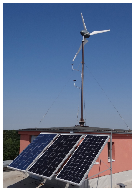
Solar-wind hybrid power plant on the roof of Lithuanian Energy Institute
