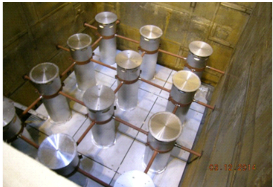
The assembly process of absorber type 1 in spent nuclear fuel pool at Ignalina NPP Unit 1
