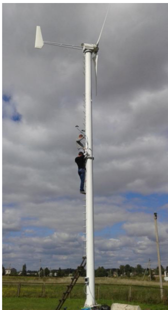
Mounting of monitoring system for wind and WPP capacity
