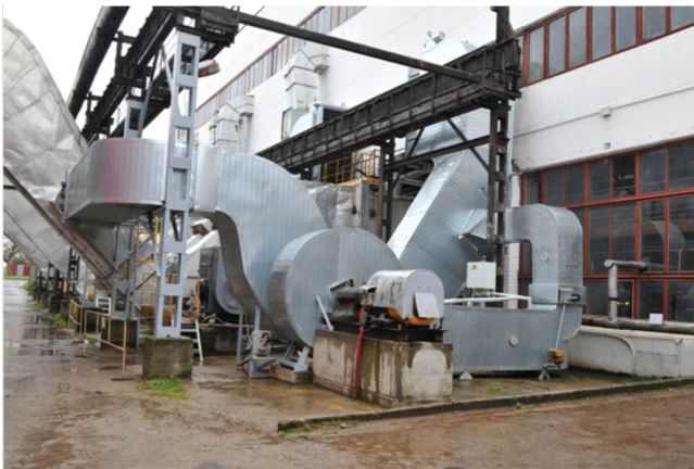
Fan and flues of flue gas recirculation system VK-5. Design boundaries and project boundaries are marked in red
