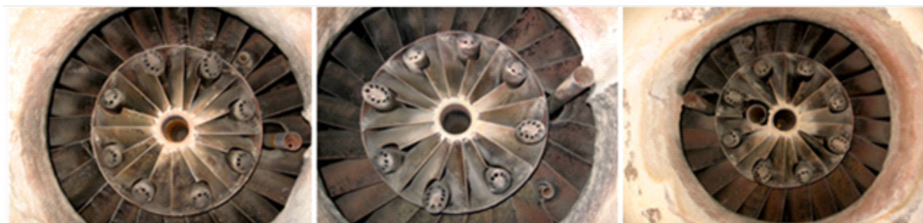
Arrangement of boiler KVGM-100 burners central and peripheral airflows and natural gas
