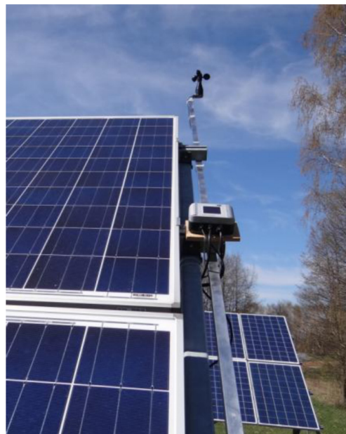
Monitoring system sensors for meteorological conditions mounted at the solar power plant
