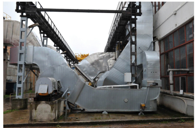
Fan and flues of flue gas recirculation system VK-5. Design boundaries and project boundaries are marked in red
