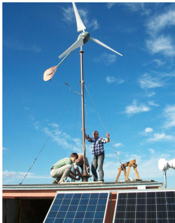
Mounting of direction stabilizer in the wind power plant on the rooftop of the Institute
