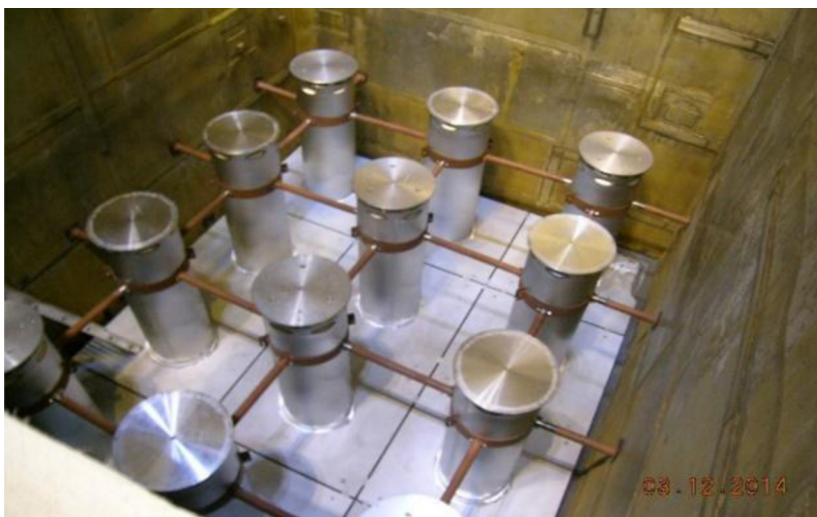
Absorbers for Ignalina NPP Unit-1 spent nuclear fuel pool
